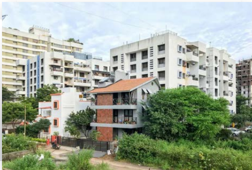
Choudhari House by M+P Architects
